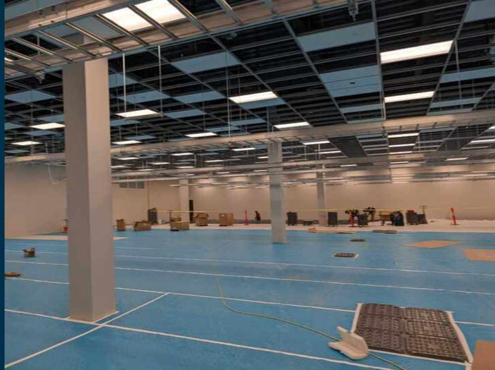
October 2025 Raised floor install
